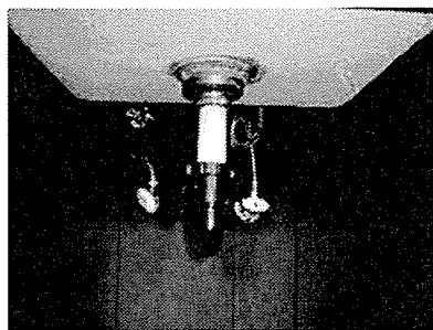
Photo #24 Asbestos containing gray undercoating sink mastic.
