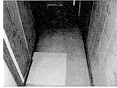
Photo #28 Asbestos containing 12"x12" light-gray tile with with white and maroon specks.
